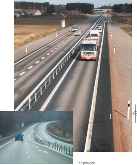
of overtaking sections every 2km reduces driver frustration and the provision of a central safety barrier eliminates imprudent overtaking. Provision for right turning movements will only be at designated junctions.
